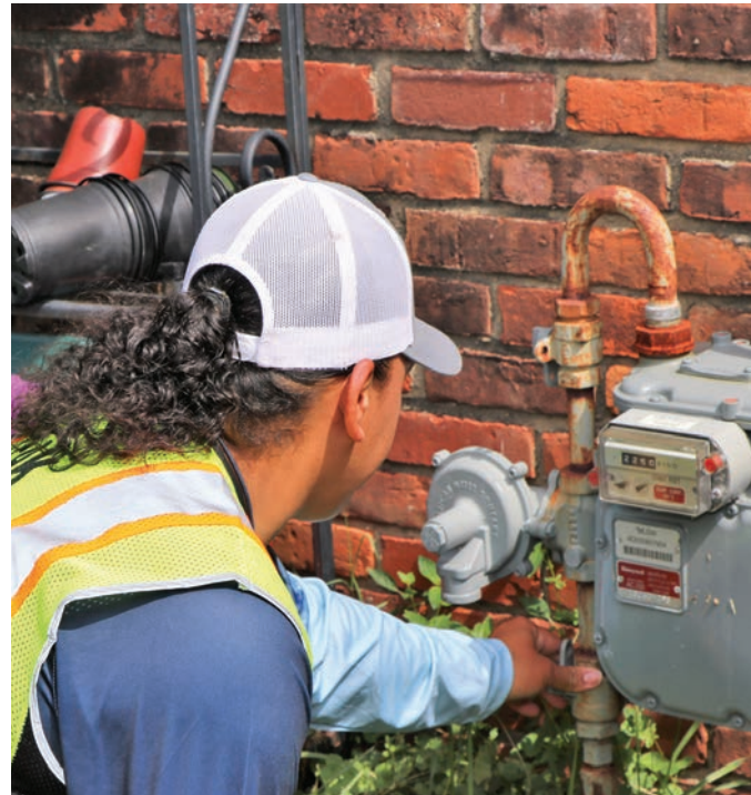
A contractor checks a residential gas meter for leaks and damages.
