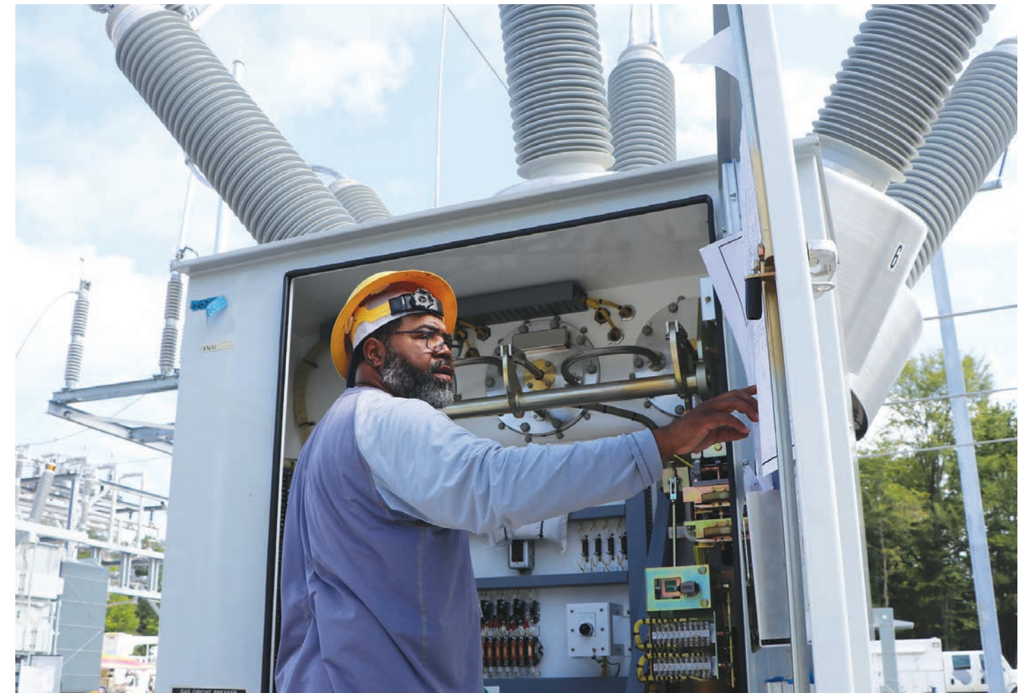
A substation ops employee checks the blueprint for a new substation.
