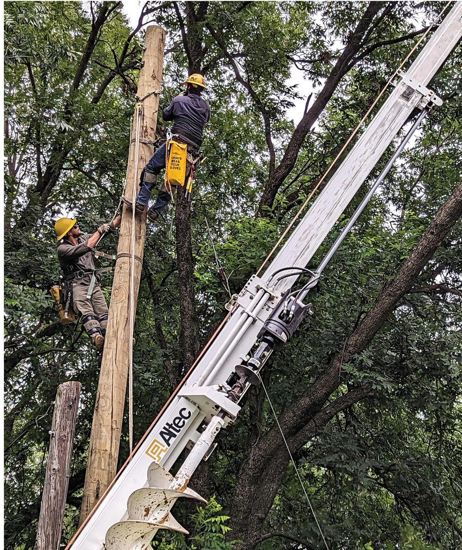
Linemen set and frame a new utility distribution pole.
