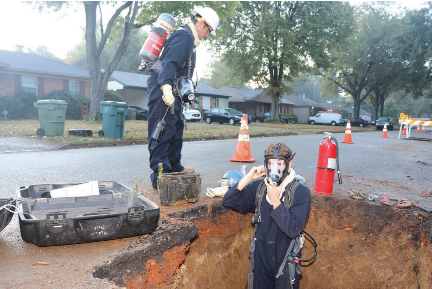
A gas worker wears a self-contained breathing apparatus as he and a co-worker set up to make repairs on a gas line. A fire extinguisher sits nearby if needed.
