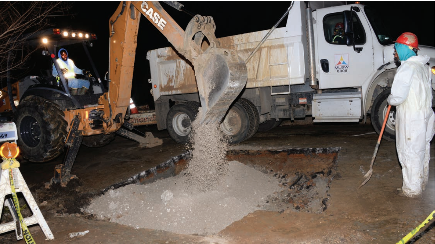
Once a water line project is completed, a Paving & Concrete Restoration crew returns to repair the street before morning rush hour.
