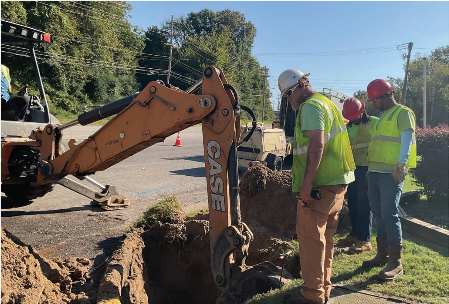
A backhoe operator carefully digs around the existing utility service lines as he replaces a water valve.
